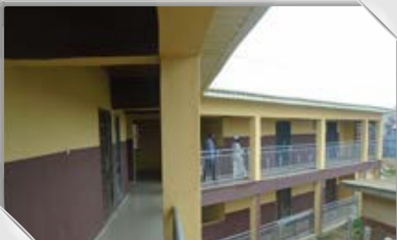
CCGG members inspecting the work done at the new reconstructed Idi-Ogunfun PHCC in Ibadan North Local Government.
